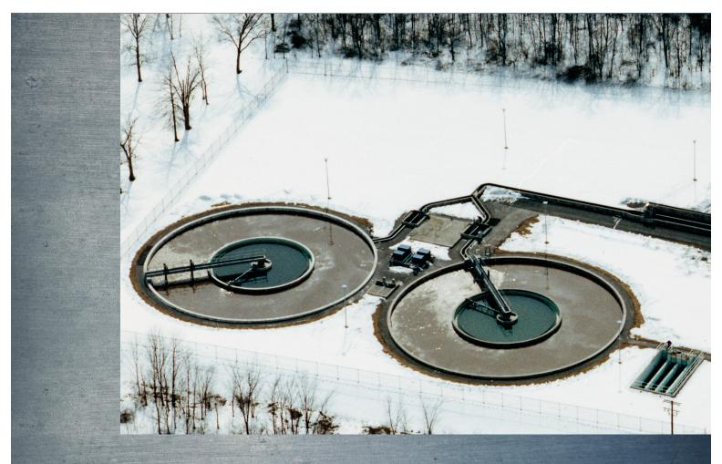
Aeration/Clarification in a single basin - suitable for ADF's up to 1.5 MGD.
