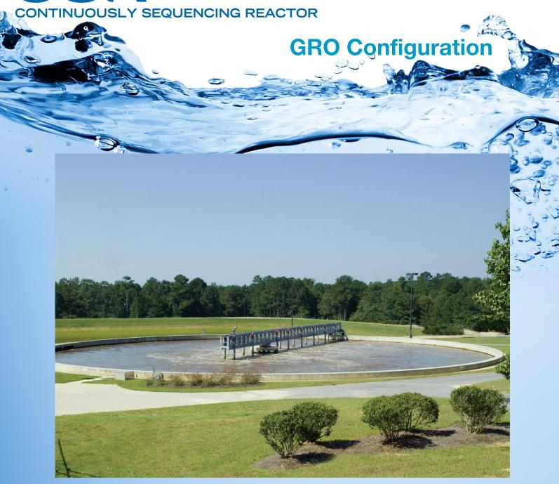
Aeration-only in a single basin suitable for ADFs from 75,000 GPD up to 3.0 MGD.
