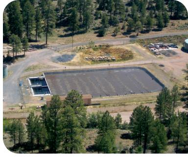
strategies using Wave-Ox<sup>TM</sup> technology (see back page) extend its capabilities to denitrification and biological phosphorus removal with no treatment basin modifications.
